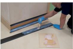
STYCCOBOND F49 can be applied to STOPGAP smoothing compounds, sound, smooth, clean, dry surfaces of concrete, sand/cement render, granolithic, terrazzo, plaster, plasterboard, flooring grade chipboard, plywood, MDF and hardboard.
