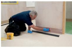
STYCCOBOND F49 can be used as a single coat pressure sensitive impact adhesive for securing PVC edging and flexible PVC skirting, coving and capping as well as PVC and PVC backed textile floor and wall coverings.
